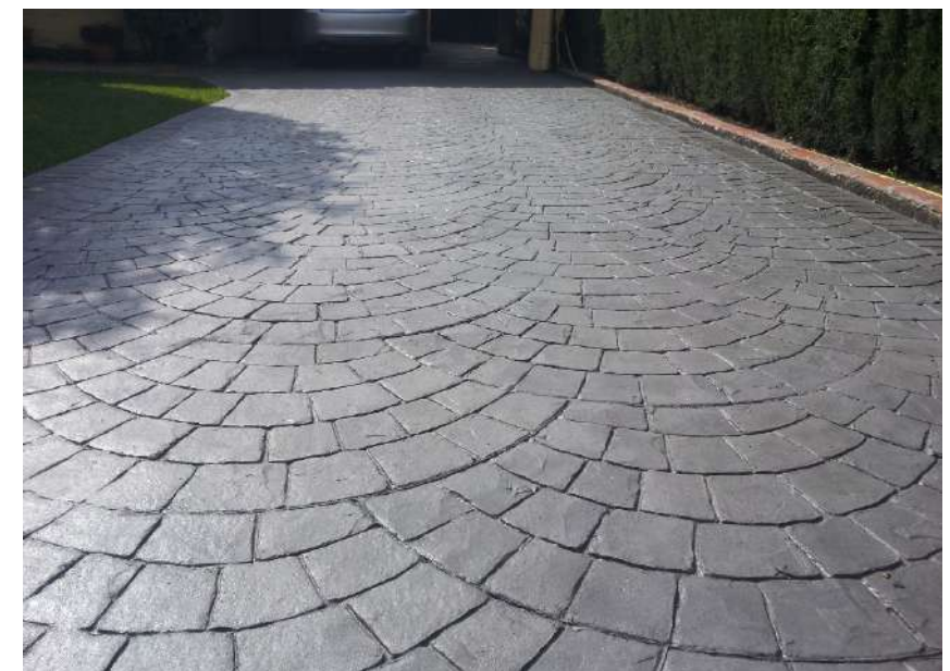
Printed concrete
